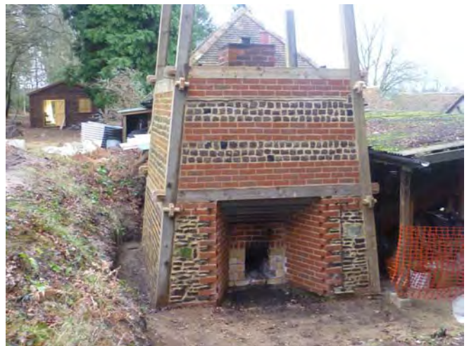
The completed furnace at Tilford (compare with the photo in the November 2011 Newsletter)
